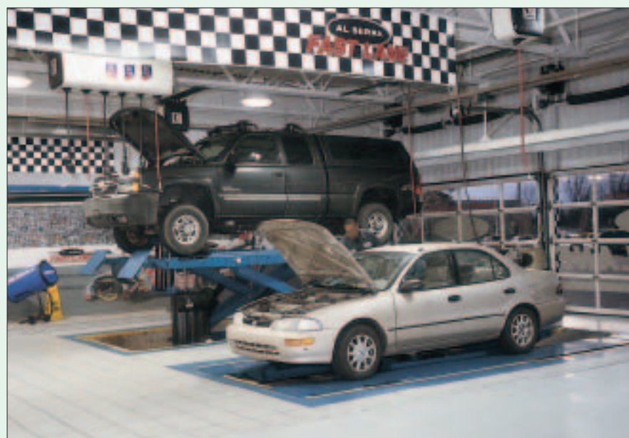
Two Hunter RX-P flush-to-floor lift racks are used to speed 15-minute oil-change service. Vehicles entering the service department through these lanes are inspected by the SS100 when exiting forward.
